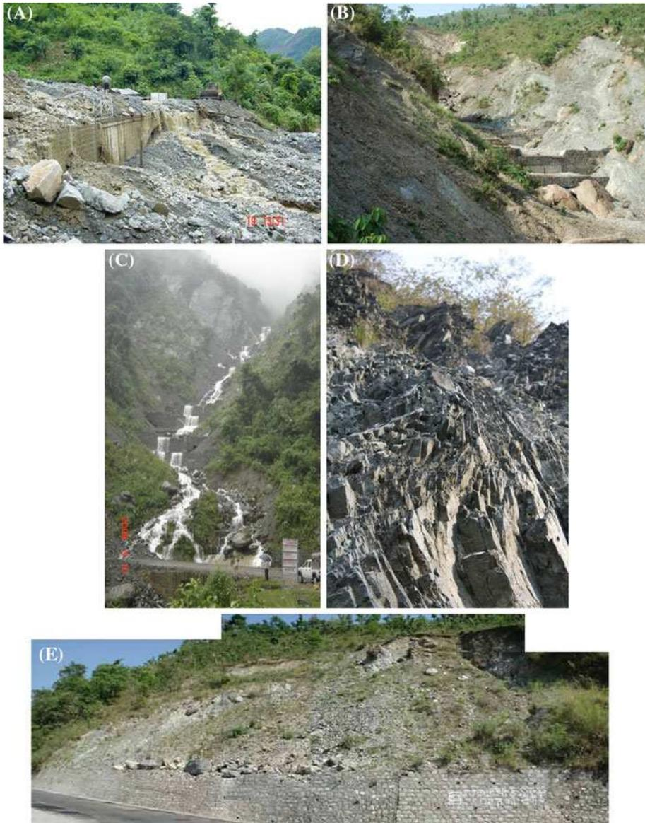
**Fig. 3** Figure showing different types of landslides observed in the study area. **a** Thick debris deposit which buried the bridge over the road section, at 21 + 500 km; **b** debris slide observed at 20 + 800 km of the road section (L2); **c** Landslide at 23 + 760 km of the road section; **d** rock topple observed at the upstream of Keraghari Khola, at 21 + 560 km; **e** slope failure observed at 30 + 500 km
